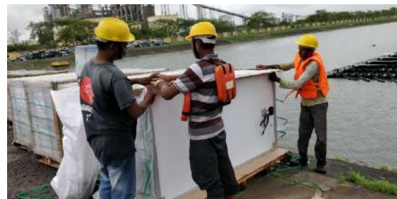
Figure 2 (a) Workers engaged in installation of floating solar PV
