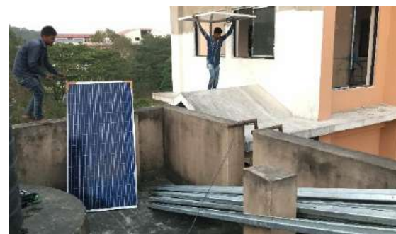
Figure 2 (b) Workers exposed to ergonomic risks while carrying solar PV panels
