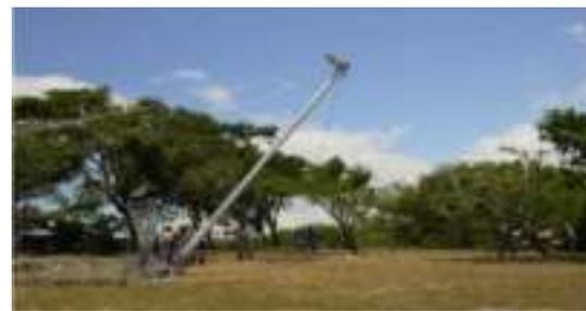
**Figure 3.6.3-7** Place box wrench in bolt holes on top of Gimbal Joint. This will keep the grip hoist cable from sliding on the Gimbal Joint during erection. Attach Grip Hoist to temporary anchor approximately 15 meters away from foundation on the opposite side from the gin pole.
