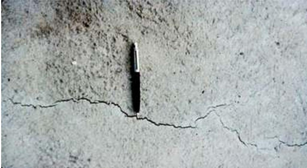
**Figure 1** A typical plastic shrinkage crack [6]
