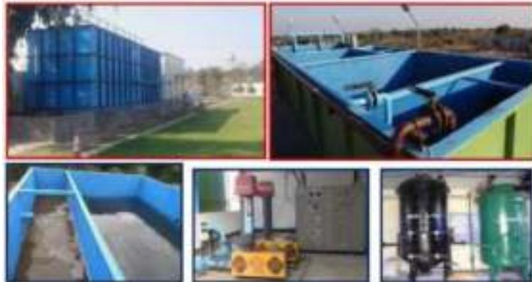
**Figure 5** New 100 KLD STP with MBBR Technology
