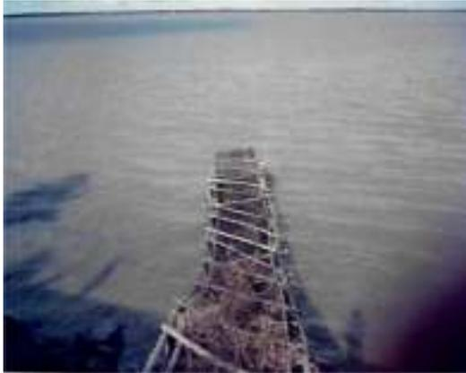
Figure 5 Semi permeable spur
