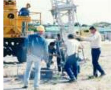
**Figure 3.6.1-4 (C)** Once the ERS Column is over the Foundation the Tie Rods on the Gimbal are released so that the bottom portion of the Gimbal can rotate. The ERS Column is lowered and the bottom flange of the Gimbal is bolted to the Foundation.
