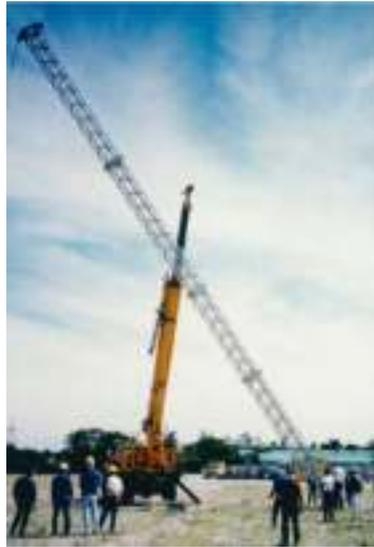
**Figure 3.6.1-4 (B)** The ERS Column and Gimbal is walked in toward the Foundation.
