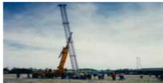
**Figure 3.6.1-5** Attach the guys to their anchors and begin tensioning. Use the guywires, not the boom, to plumb the column. After the guys are installed the winch line can be slacked off.
