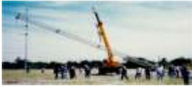
**Figure 3.6.1-4 (A)** The ERS Column is picked slightly above the center of gravity. The ERS Column is raised directly over the foundation
