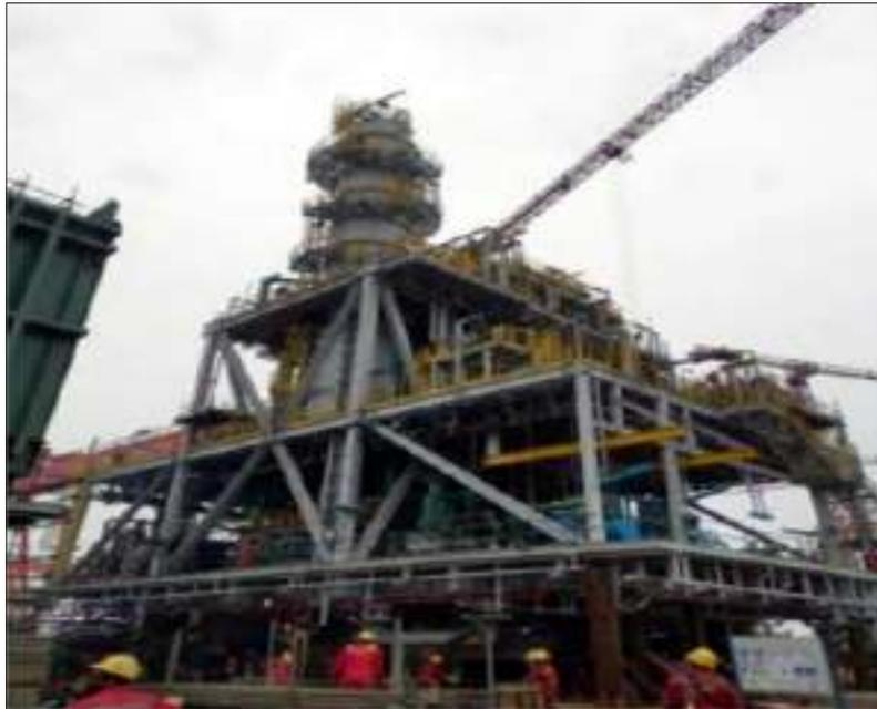
**Figure 5** Module with conventional deaeration tower
