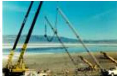
**Figure 3.6.1-1** Erecting an ERS with two sets of cranes. One crane lifts the top and one crane moves in the Foundation.
