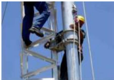
**Figure 3.6.3-15** Hand tighten then tighten with wrench.
