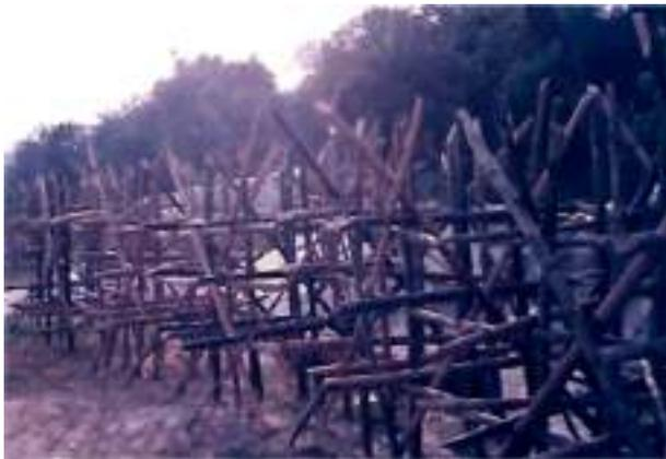
**Figure 3** Bamboo porcupines (making in progress)
