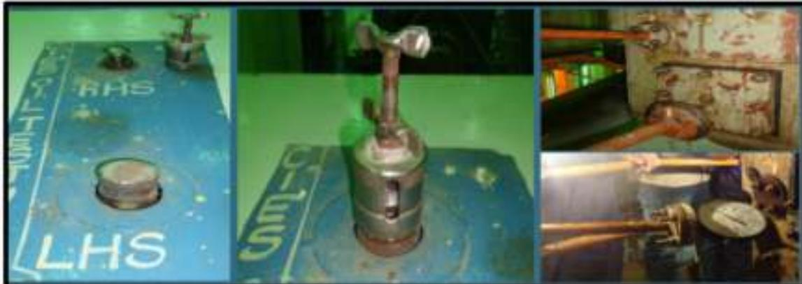
**Figure 2** Gag for CIES valve (RHS) onload test valve
