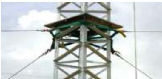
**Figure 3.6.3-20** The slings must go around one or more of the 3" x 3" (76 mm x 76mm) main vertical angles.
