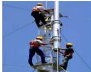
**Figure 3.6.3-16** Lift the Gin Pole Mast
