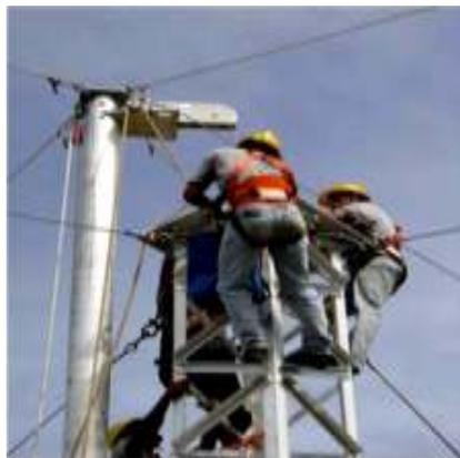
Figure 3.6.3-11 Note the positioning ropes on the gin pole, four places used to keep gin pole centered when lifting.
