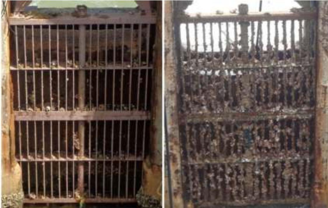
**Figures 1 (a)** AFC applied screen **(b)** Non-AFC applied screen
