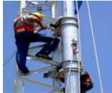
**Figure 3.6.3-14** Turn the slider and close the swing clamps around the large angle.
