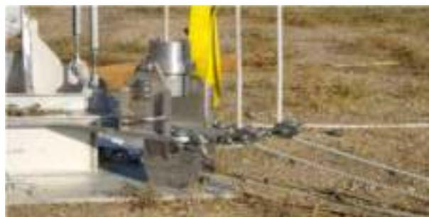
**Figure 3.6.3-18** Gin Pole Tilt Up Hinge
