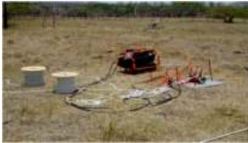
1. Place capstan 20 to 25 meter from foundation inline with gin pole.
