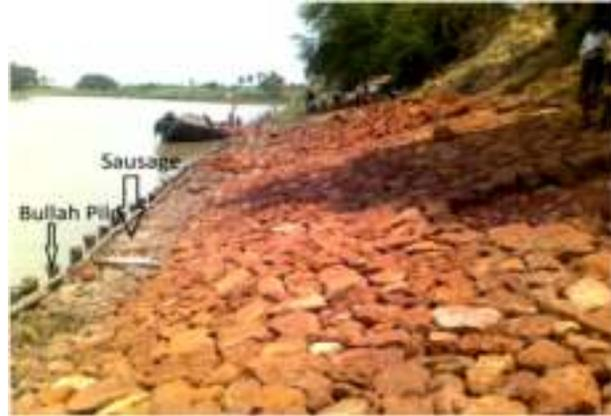
Figure 6 Sausage used to protect embankment
