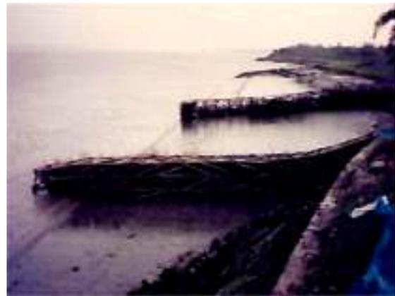
**Figure 4** Semi permeable spur
