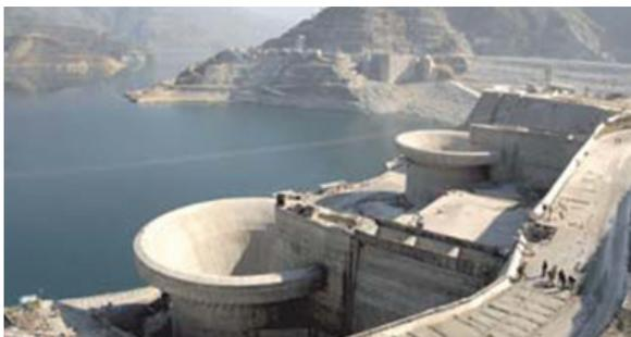
Figure depicts the Right Bank Morning Glory Shaft Spillways (ungated) with top at FRL El. 830.00 and the section indicates right Bank morning glory spillway showing Intermediate Level Irrigation Outlet
