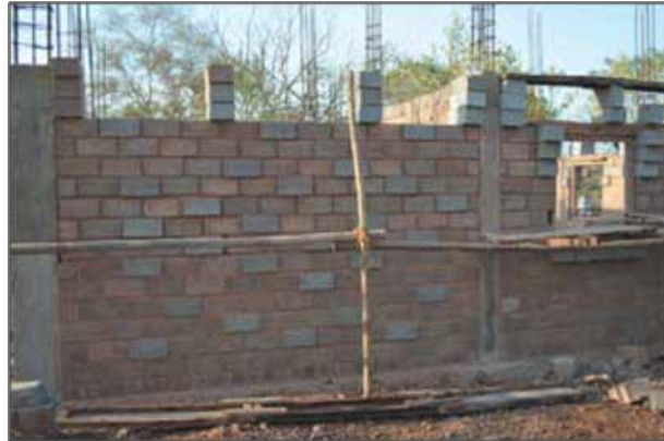
Fig. 11. Construction of two story house using LC 3 [14]
