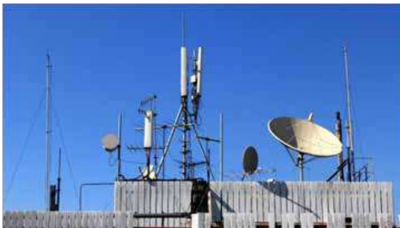
Fig. 2. Multiple antennas closely mounted at control station
