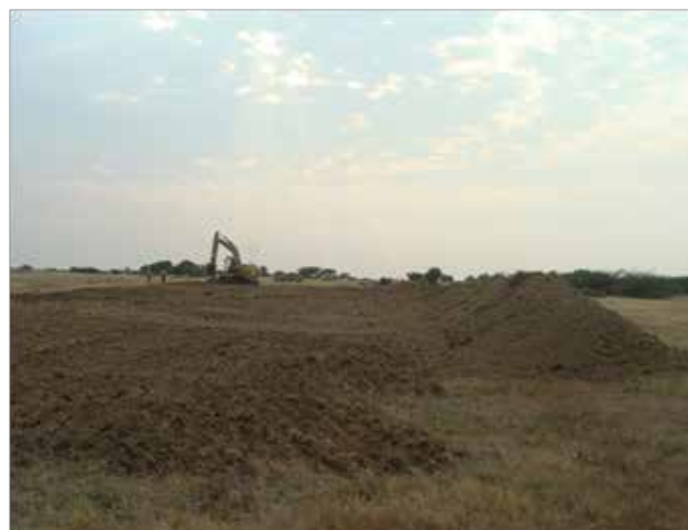
Fig. 1. Stripping of topsoil
