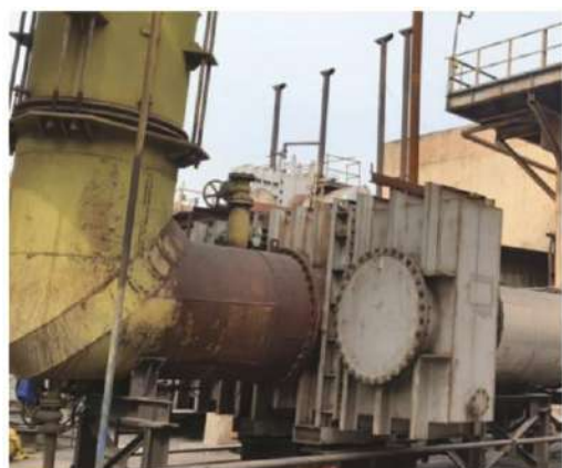
Figure 2 Typical installation of Goggle Valve in gas piping main.
