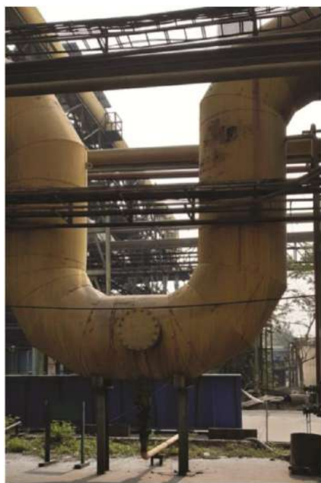
Figure 3 Typical installation of U Seal in gas piping main.
