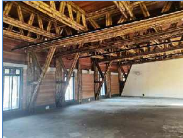
Figure 3 Truss configuration
