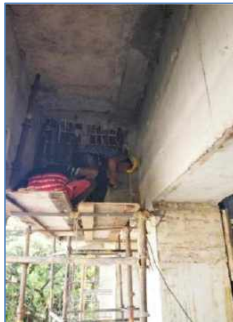
Figure 5 Drawing of Exposed Shear Reinforcement.
