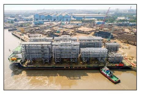
Photograph 2 Modular plant being transported, at loading port of LTEH, Hazira
