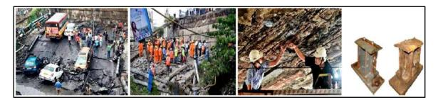
Figure 1 (a)-(b) Catastrophic failure of bridges, (c)-(d) Distress in bridge deck slab and bearings [4]
