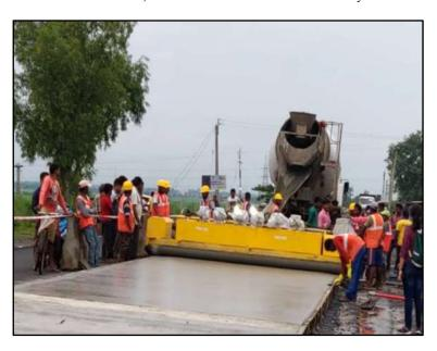
Figure 1 Construction process of Whitetopping
