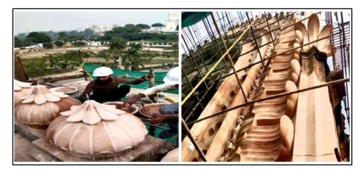
Images 3A & 3B Stucco work, design moulding work, highly rich intricate plaster work in traditional lime mortar with natural adhesives
