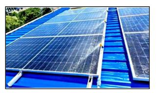
Figure 1 Semi-automated cleaning under progress of the solar PV power plant
