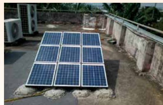
Nine Solar panels connected together to form an array
