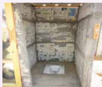
Semi-finished assembly of precast slabs for toilets
