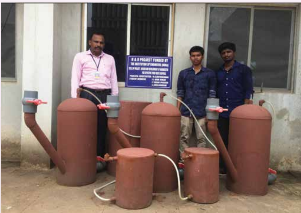
Biogas digester plant setup installed in Men's Hostel of Saveetha Engineering College, Chennai to generate cooking gas from food waste
