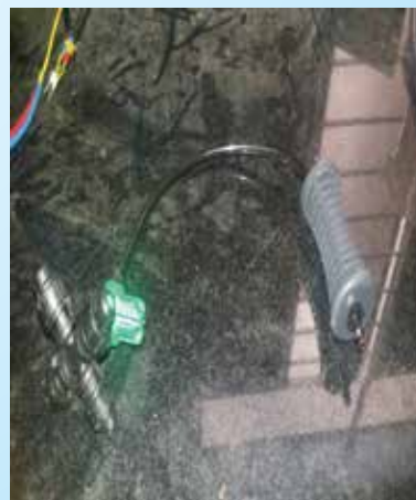
Nozzle used for mist formation in the condensing coil
