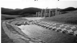
Channel Type Fish-way
