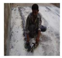
Photo 13: Thermosealing of the joints
