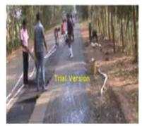
Photo 15: Application of tack coat before laying BJPF
