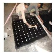
Photo 12: Placing of antiskid stone chips on masticated surface
