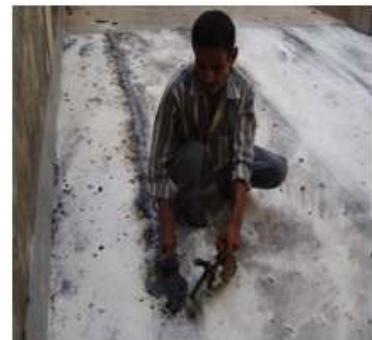
Photo 13: Thermosealing of the joints
