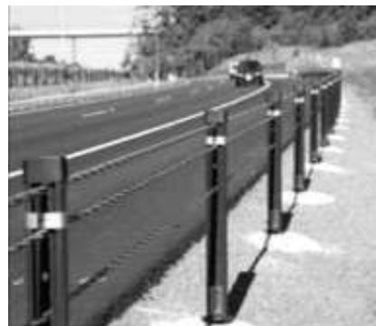
Figure 7: Wire rope safety barriers for minimizing impact
