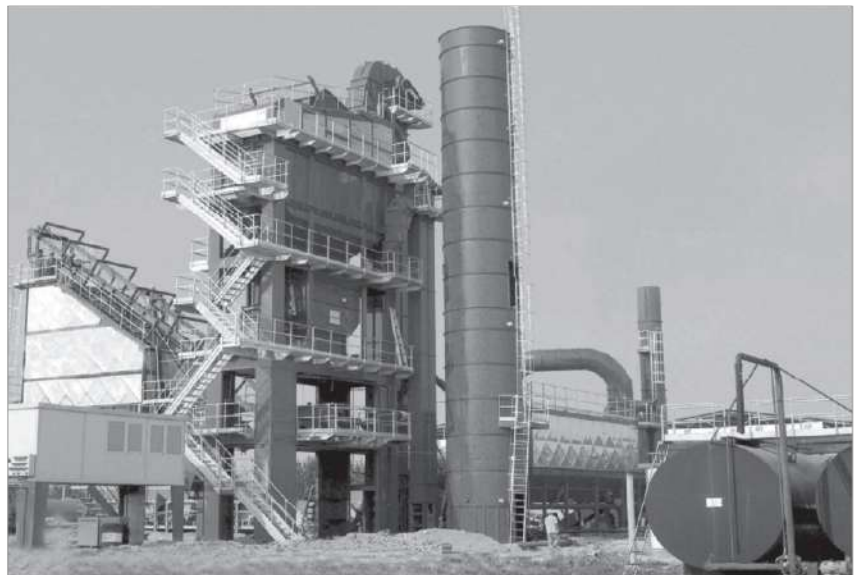
Construction site of a plant
