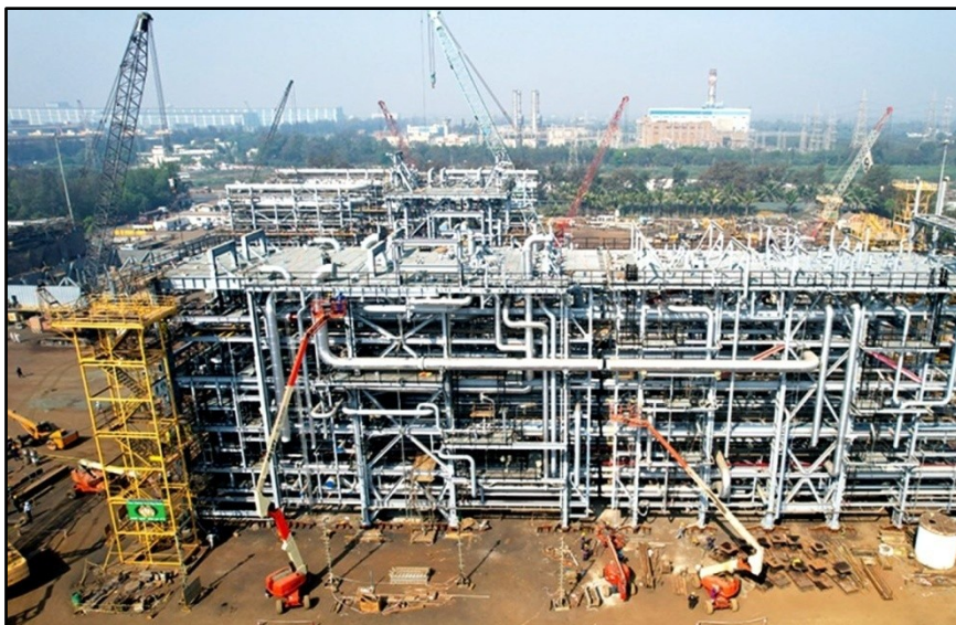
Photograph 1 LTEH (L&T, Energy and Hydrocarbons) MFY (Modular Fabrication Yard) at Hazira
