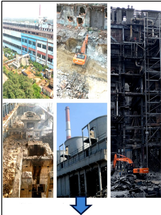
Figure 1 BTPS Main plant dismantling snapshots
