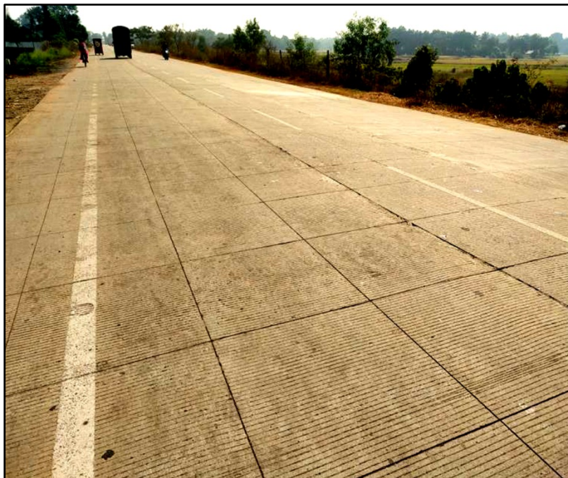
Figure 2 Constructed Whitetopping road in operation
