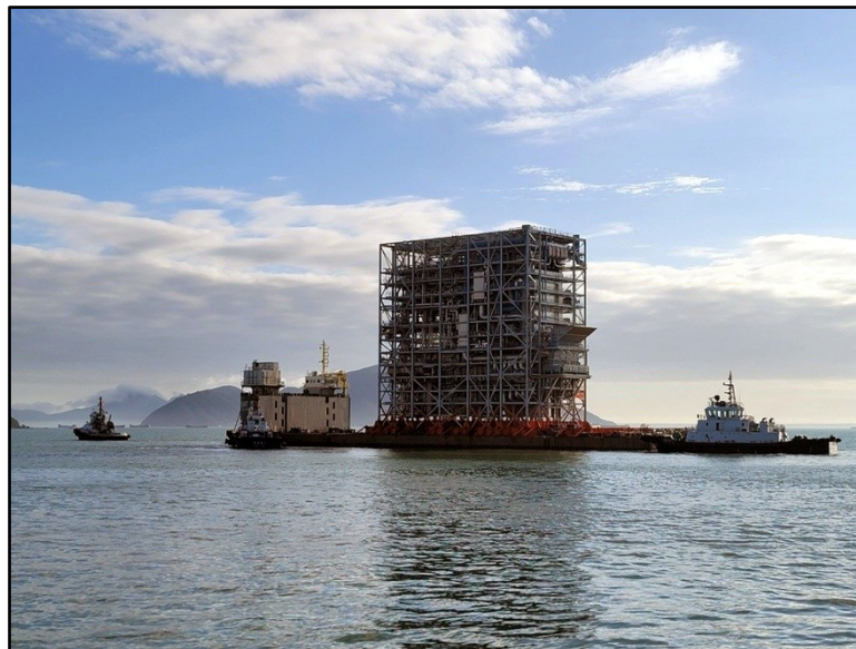
Photograph 3 Typical modular plant being transported, in transit
