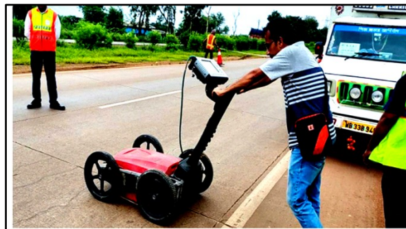
Figure 1 GPR Scan being conducted on the study stretch
