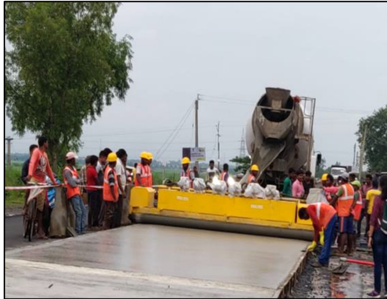
Figure 1 Construction process of Whitetopping
