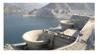
Figure depicts the Right Bank Morning Glory Shaft Spillways (ungated) with top at FRL El. 830.00 and the section indicates right Bank morning glory spillway showing Intermediate Level Irrigation Outlet
