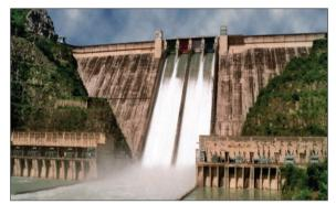
Two power plants are located on either side of the spillway d/s of the toe of the dam. There are two canal power houses in the Nangal Hydel Channel, and the total installed capacity of Bhakra Nangal System is 1354 MW. The Bhakra dam feeds a network of irrigation canals which command an area of 2.63 MHa in the states of Punjab, Haryana & Rajasthan, in addition to stabilizing and improving irrigation under three existing canal systems.
