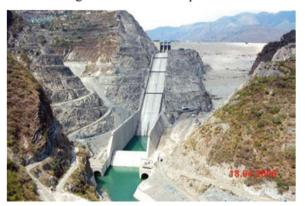
Figure: A perspective view of Chute Spillway with three Crest Gates, located on the right bank hill slopes (in deep cut sections, to found them on competent fresh rock and also to satisfy the desired hydraulics for ensuring smoother transitions)
