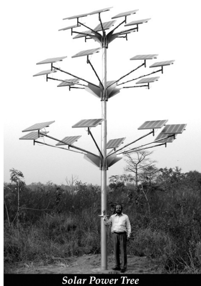
Figure 3 : Prototype of solar power tree (tall 9.144 m) capacity 2.5 kWh (max)
