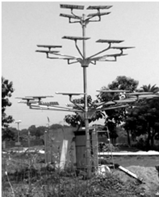
Figure 12 : Solar power tree - a tall single trunk with multi-stage branches
